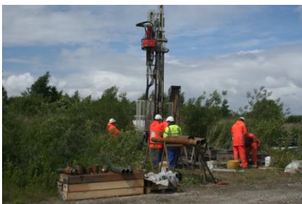
Appreciate the skill of rock drilling for good coring
